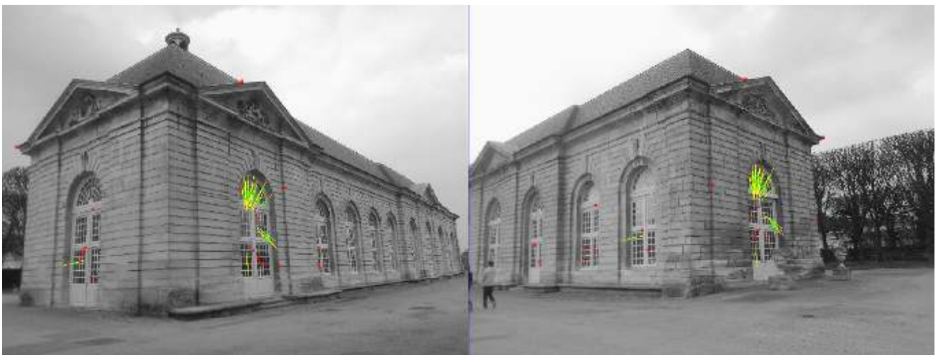
Figure 8: Incorrect estimated model between different facades of the Orangerie de Sceaux, with a threshold of 1.1 pixel.
